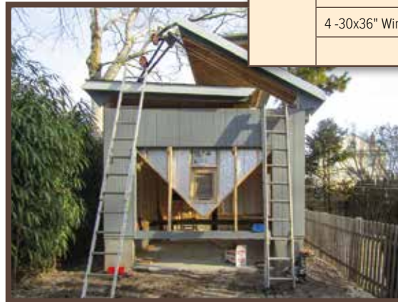
Jacking up Roof
