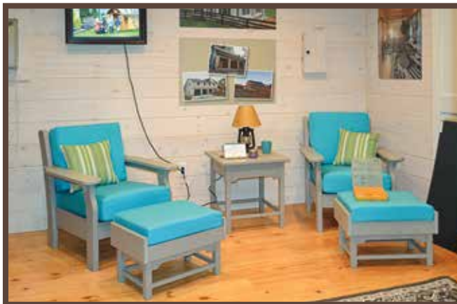
Finished Interior Tongue and Groove Pine
