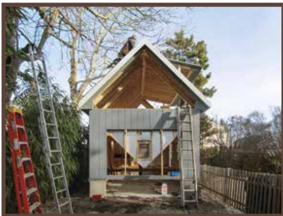
Hinge Roof Under Construction
