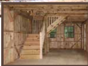
Rough Cut Oak Framing
